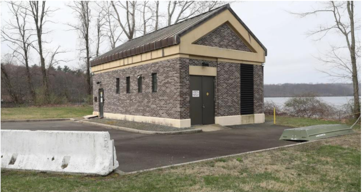
The pump station at the Westchester Joint Water Works in West Harrison, April 9, 2021. Mark Vergari/The Journal News
