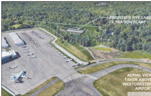
An aerial view of the location of the Rye Lake Water Filtration Plant adjacent to Westchester County Airport.
