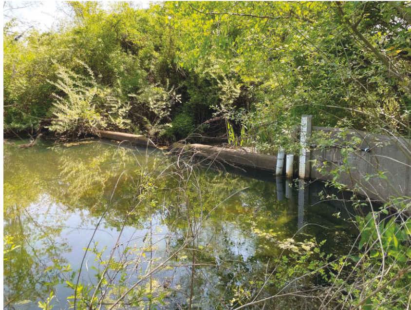
Figure 2: Existing Extended Detention Basin Outlet Weir
